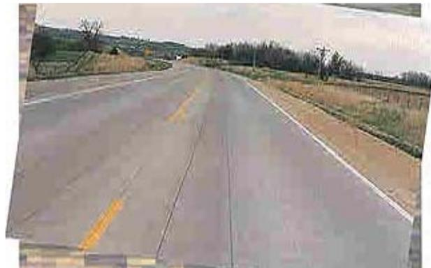
Researchers began to ask: "What if we reduced the thickness of the whitetopping... reinforced the material... and reduced stresses by redefining joint spacing requirement?" *The result: Ultra-Thin Concrete Whitetopping.* And these days, UTW is the ideal solution for city streets and intersections... local or low-volume roads... parking lots... even general aviation applications such as taxiways, runways and aprons. It bonds to the asphalt surface and works like concrete pavement!
